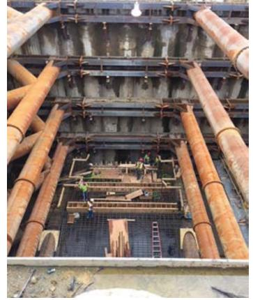
This photo shows the secant piles and temporary steel holding back the lake.
