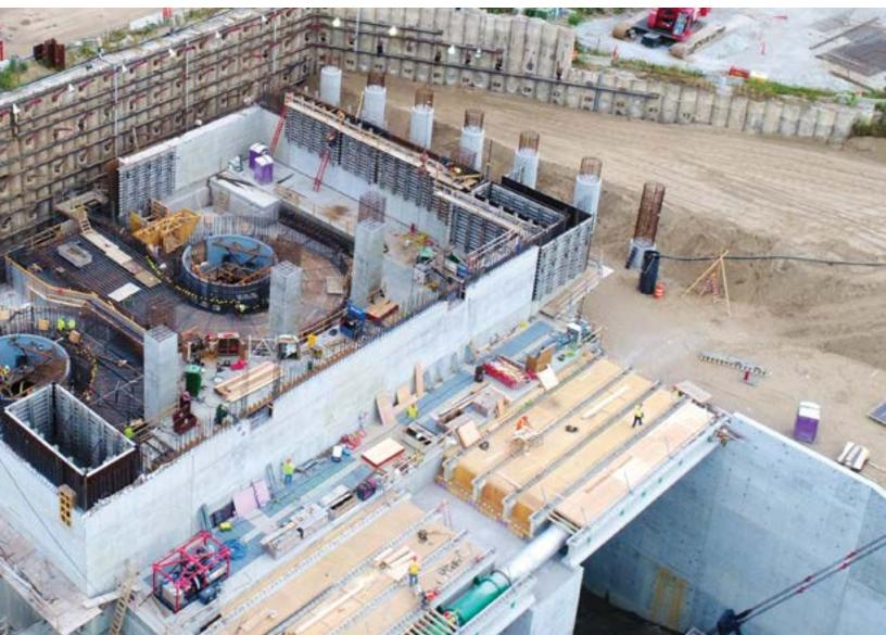
Two 21-foot-diameter penstock pipes will connect the powerhouse structure to the intake structure on the reservoir side of the dam. The steel penstock liner will be embedded in concrete and feed the powerhouse with 14,000 cubic feet of water—equivalent to 2,456 standard bathtubs full—per second.
